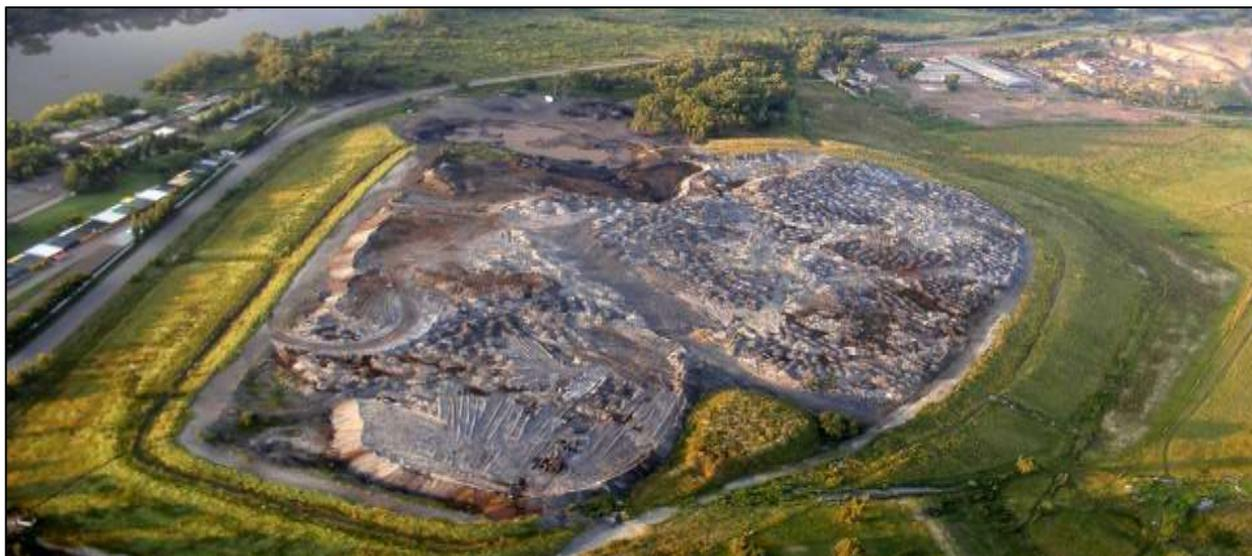
Photo 5 Capping layers on side walls and vegetation growth
