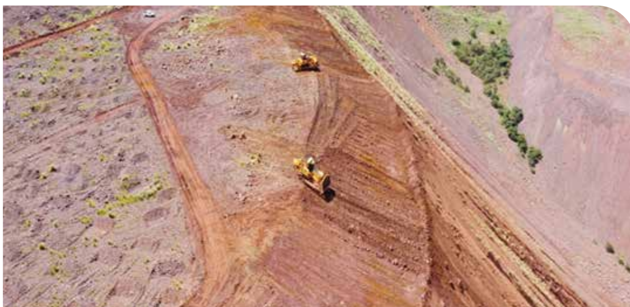
To improve safety, bulldozers undertaking potentially hazardous reshaping work at Thabazimbi iron ore mine are operated remotely.
