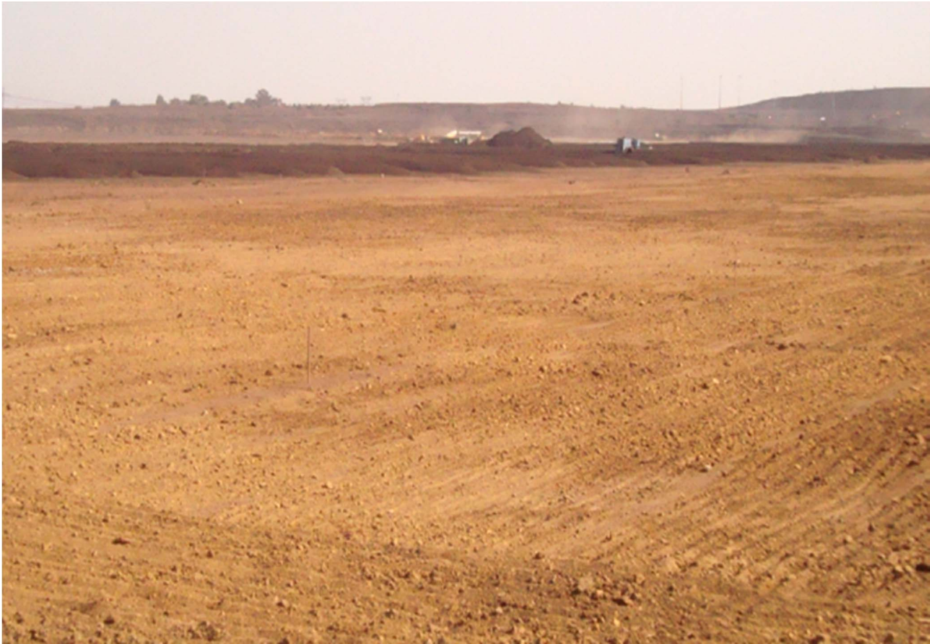
Rehabilitation in progress
